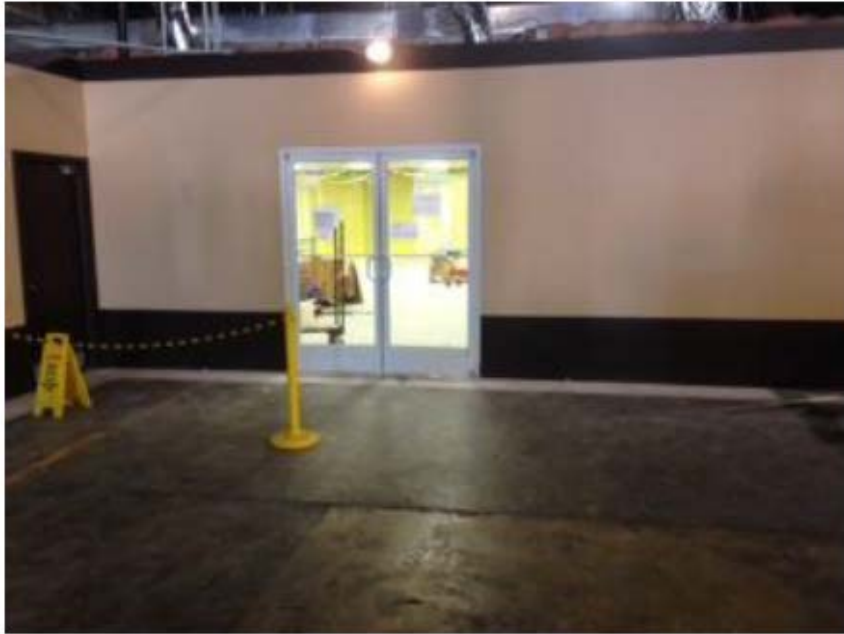
Exterior During Construction
